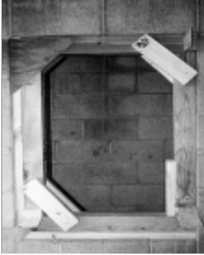
Window Shore In Masonry wall
